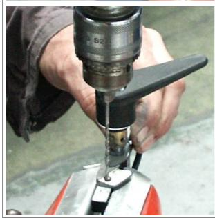
Make a small dimple using drill bit  $\emptyset$  2.4 mm to mark position of screw hole on the handrail. Dimple position must be in the center of hole through locking hook.
