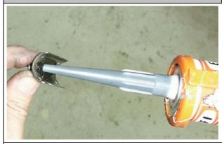
Apply Emfimastic PU 50 (or equivalent) on the inner side of the new supplied upper pin.
